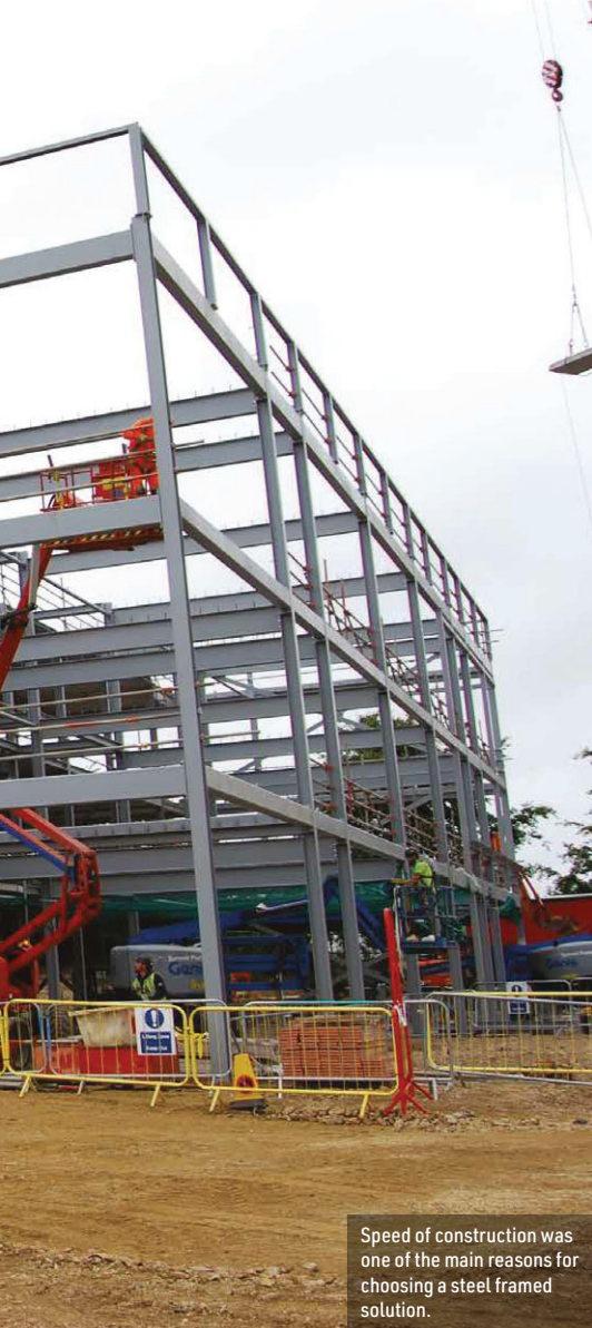
As the ground is generally good, steel columns have been installed on pad foundations.
