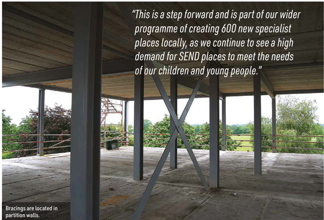
As the ground is generally good, steel columns have been installed on pad foundations.
