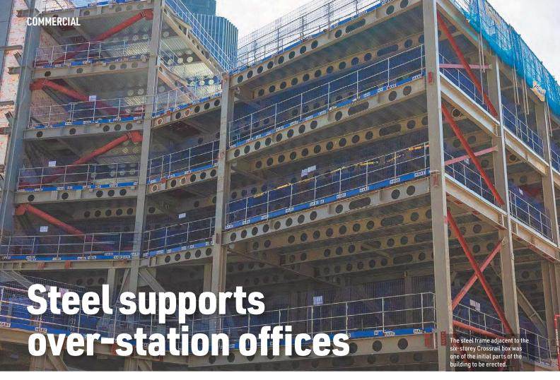
Forming a bridge over underground railway assets, a series of large steel trusses are enabling the construction of a new City of London commercial development.
