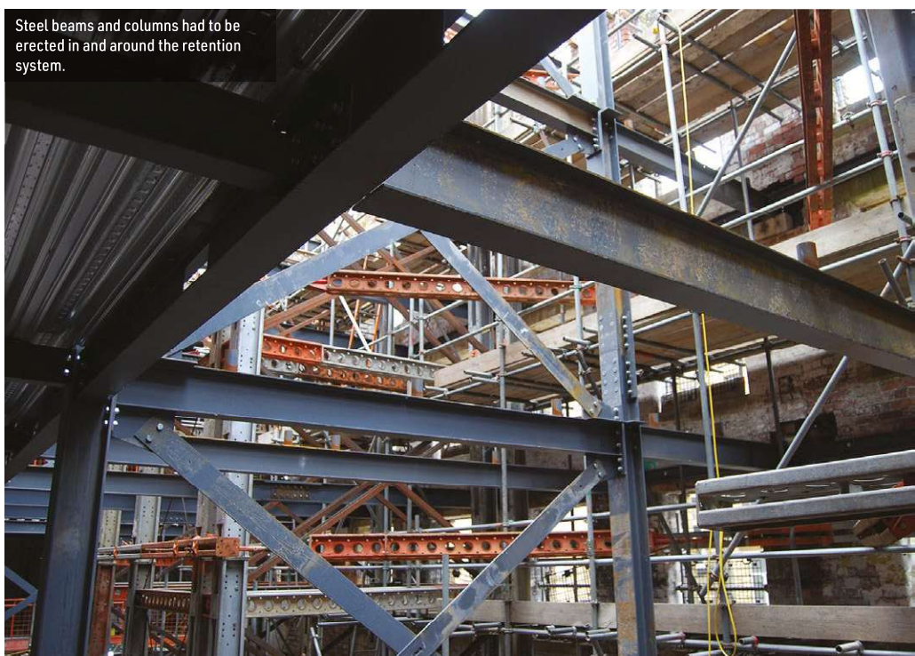
A retention system, which supports the existing façade, will be removed once the new steelwork has been installed.
