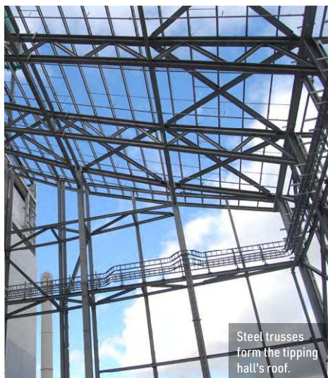
The steel-framed facility is nearly 200m-long and reaches a height of 54m.
